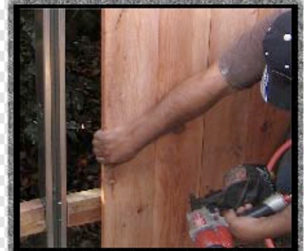
NAIL ON FENCE BOARD
